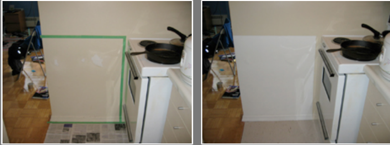
Before and after the paint.
